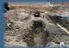
Figure 1: Protective Sleeving to Pile Locations
